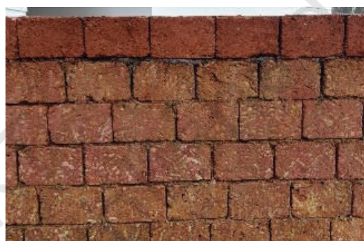
Fig. 11.7: Laterite rocks used as bricks
