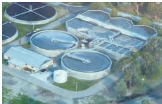
Figure 8.7 An aerial view of a sewage plant
